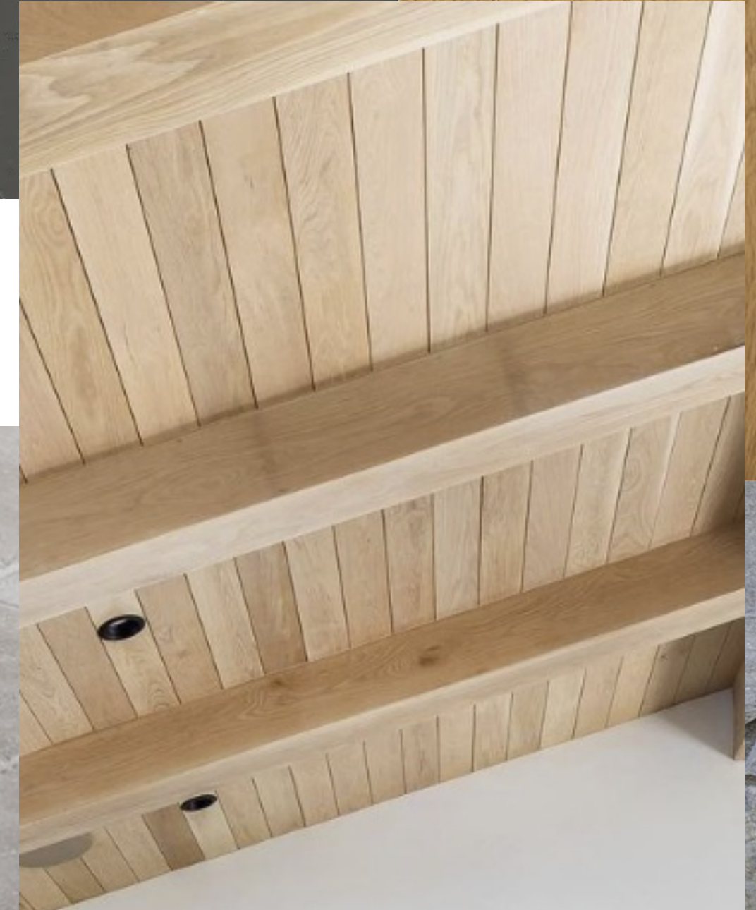
Wood Ceilings + Beams
